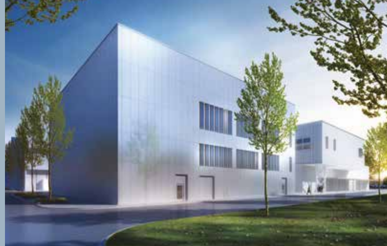
Foundations laid — A test center for engine components is currently being built at MTU in Munich.
