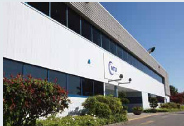
Variety _____ In addition to an engine test bench, MTU Maintenance Canada also possesses test cells for accessories such as actuators, fuel pumps and starters.
